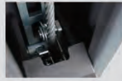
Protective device for slackening steel ropes
